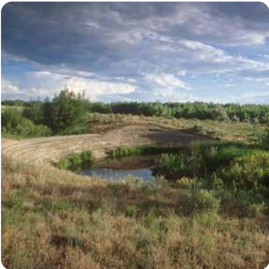
A series of stilling basins to treat stormwater runoff
